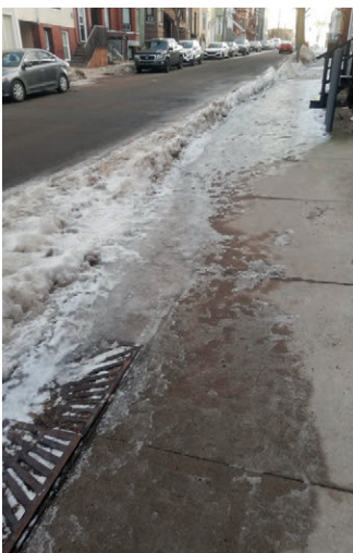
◀ Figure 10: The conditions after an ice storm can be extremely hazardous for pedestrians and motorists (Photo: ACAP Saint John).
