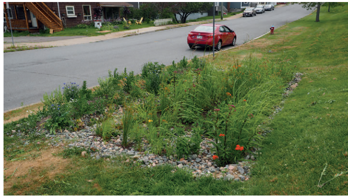
◀ Figure 18: In 2019, ACAP Saint John installed a rain garden on Queen Square West as a pilot project for the City. Green infrastructure can include implementing rainfall capture systems, permeable pavement, green roofs, bioswales, and rain gardens (Photo: ACAP Saint John).
